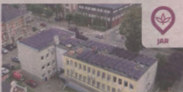
530 paneli o mocy 175 kWp
